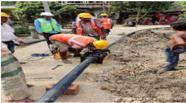
Partial use of PPEs seen at zone-15 (Pipeline)
