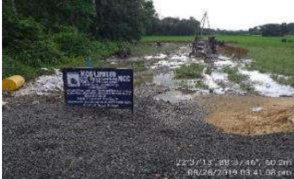
Partial water logging and improper storage of construction material at zone-12(OHR)
